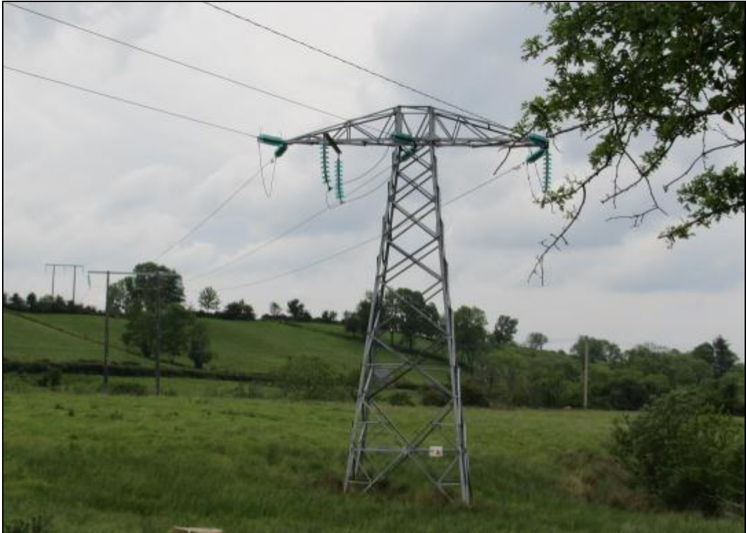
Figure 8.9: Photograph of a 110 kV Non-Earthwire Angle Mast
